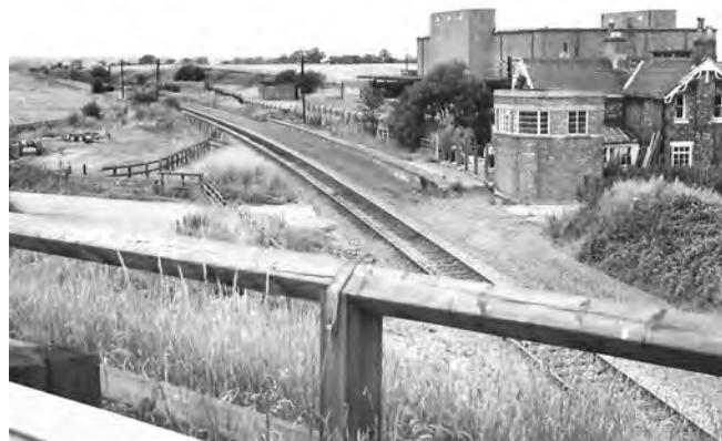
The Goldsborough cold store in the mid-1970s showing the proximity of the connecting railway line. Photo John L Smith
